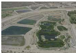
City of Tucson Sweetwater Recharge Facility
