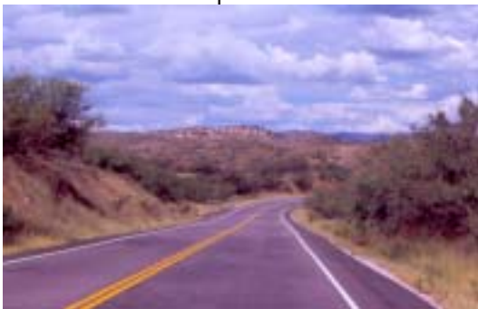
Existing road conditions
