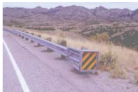
Existing guardrail along the Scenic Road
